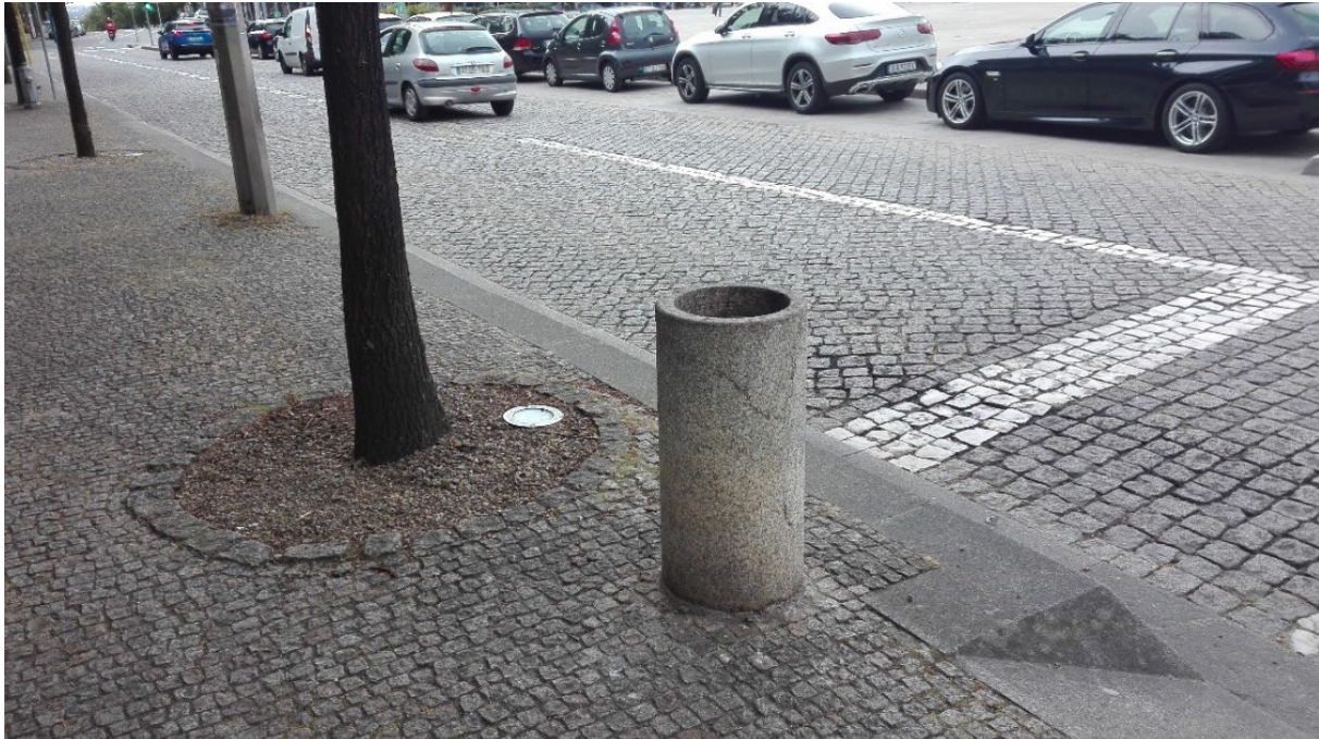
Figure 11: Installation of floodlights in the tree pits
